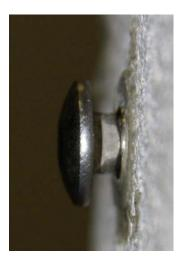
If your system has the bolts removed and the inserts are secured with covers, remove the covers and install the carriage bolt. Screw down to within 1/8" of the surface. Slide the clip over the bolt and snug down the strap.
